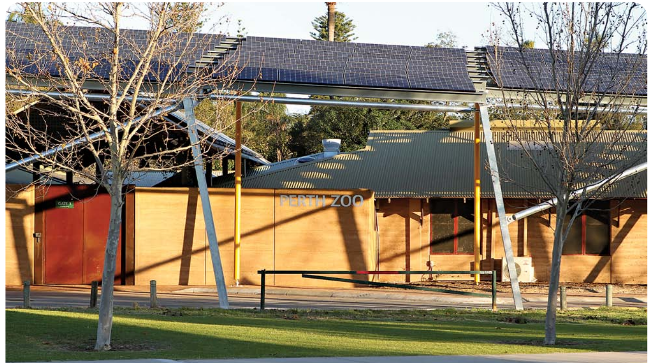
Solar installation at Perth Zoo
